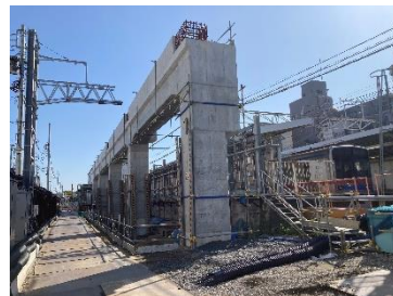
Work to construct elevated section: Near Keisei-Tateishi Station
