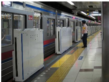
Platform doors being installed at Oshiage Station
