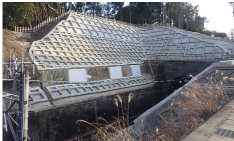
Slope reinforcement work (between Sōgosandō Station and Kōzunomori Station)
