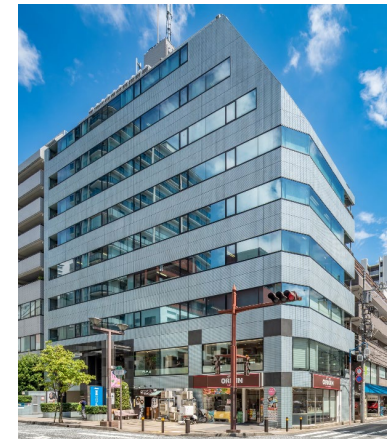
Keisei Minami-Yawata Bld. (acquired in Nov. 2022)
