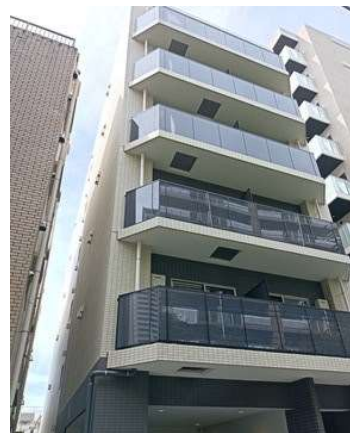
Skygrande Ichikawa (completed in Aug. 2022)
