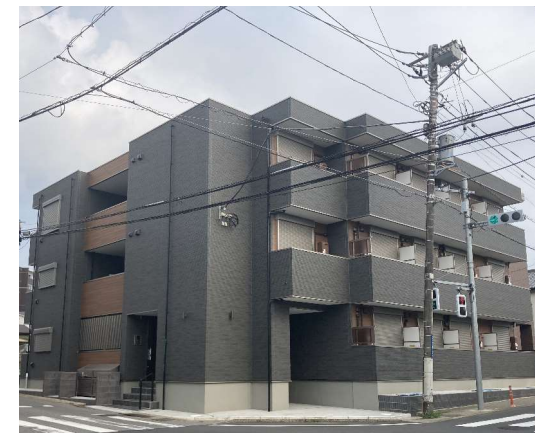
Windterrace Yachiyodai-nishi (completed in Aug. 2022)
