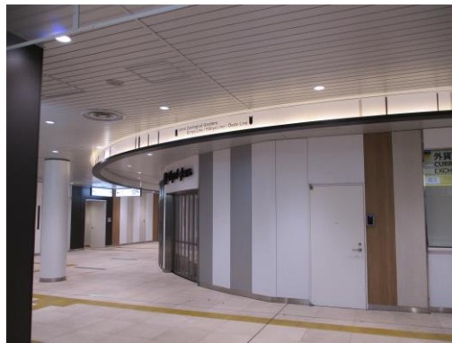
We're rolling out LED lighting
