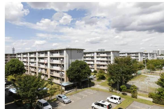
Sodegaura housing estate (source: Urban Renaissance Agency)
