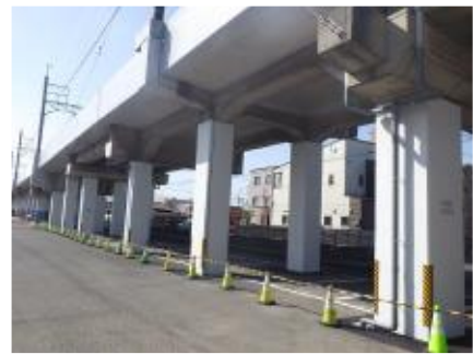
Track elevated for better earthquake resilience
