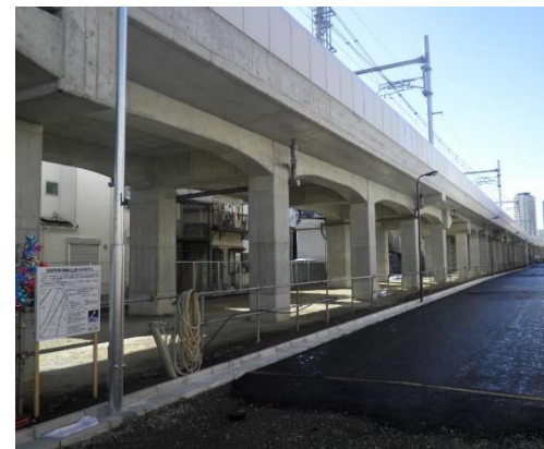
We're elevating the Oshiage Line (the photo shows a section in Sumida-ku)
