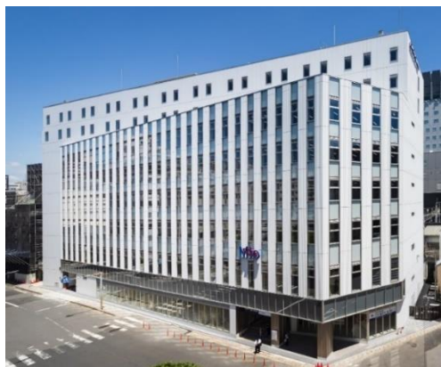
The Keisei Chiba-Chuo building was recently rebuilt
