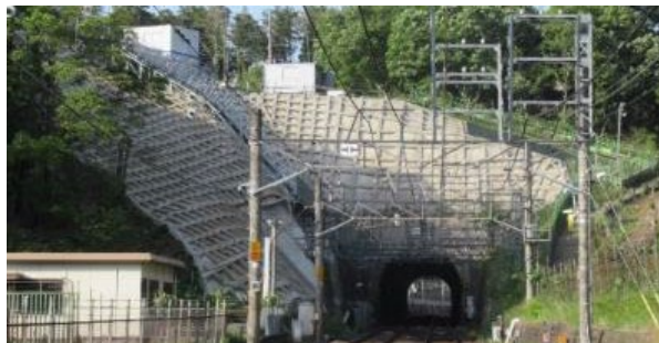
Slope reinforcement (Sogosando Station – Kozunomori Station)
