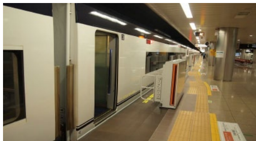
Platform doors installed at Narita Airport Station
