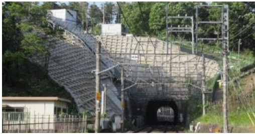
Slope reinforcement (Sogosando Station – Kozunomori Station)
