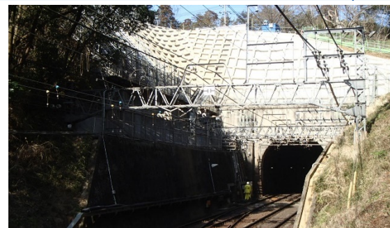
Reinforced slope between Sogosando Station and Kozunomori Station
