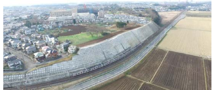
Reinforced slope between Usui and Sakura
