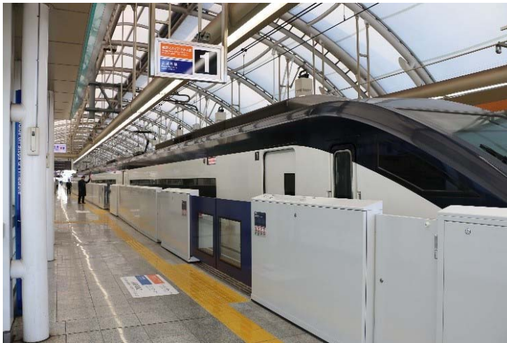
Platform doors (photo: outbound platform, Nippori station)
