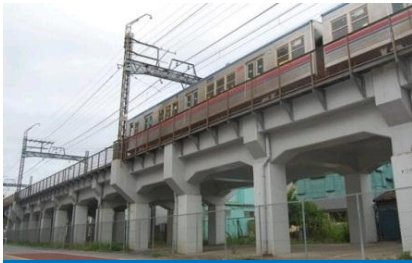
Seismic reinforcement for elevated railway tracks
