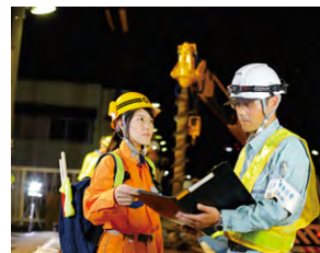
Female employee working at a construction site
