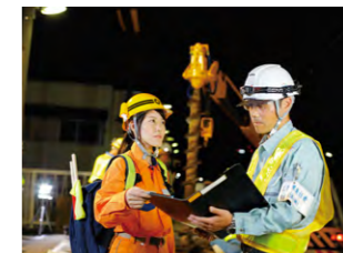
Female employee working at a construction site
